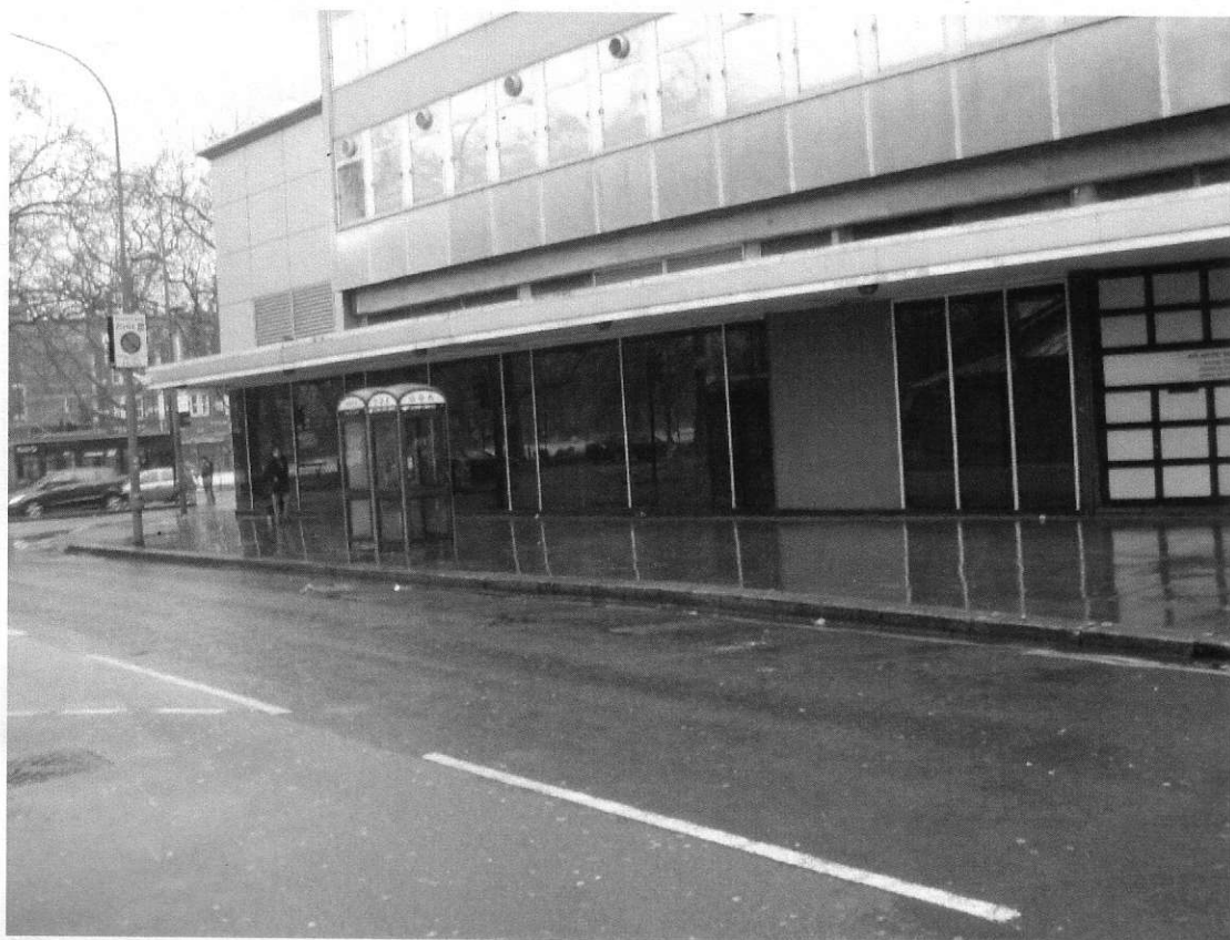
Picture showing a distinct absence of a time plate outside number 1 Rockley road.
